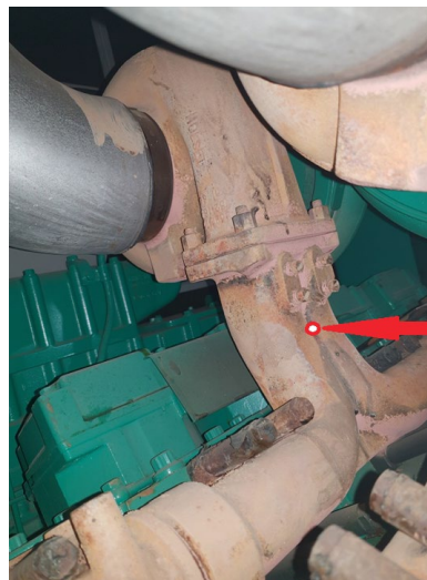
FIGURE 14 MARK WELD-IN BUNG PLACEMENT
